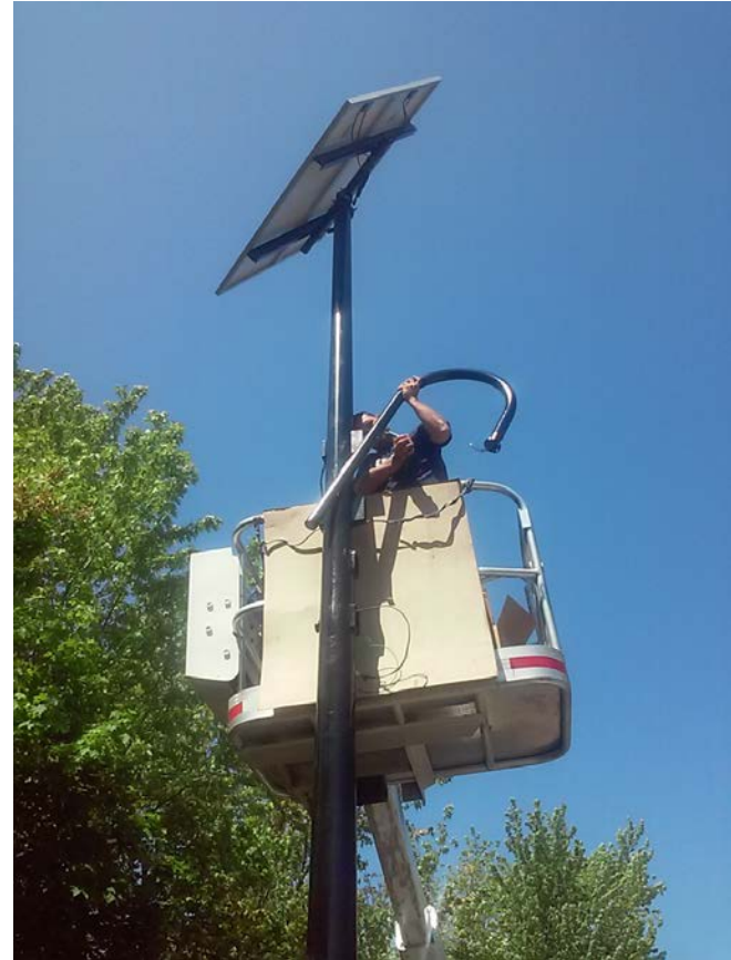
City of Somerville workers helped install the SolarOne LED lights
