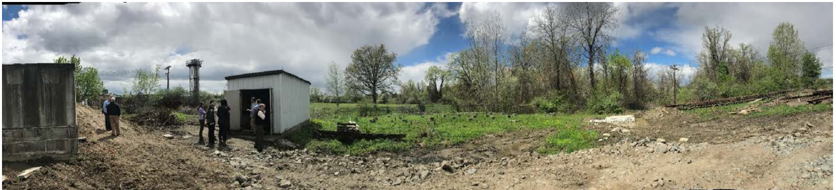
Amherst Wastewater Treatment Plant and Clean Membranes Pilot Site
