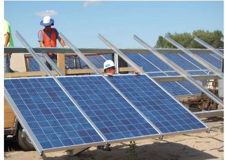
Construction of the CES Vineland Solar Site – August 2011
